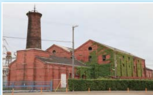
No.1 Boiler at the Aboshi Plant
